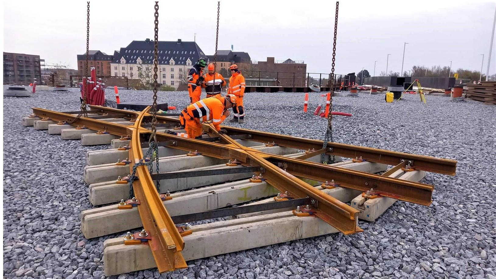
Switches will be installed on the ramp leading the Light Rail to and from Glostrup Station.
